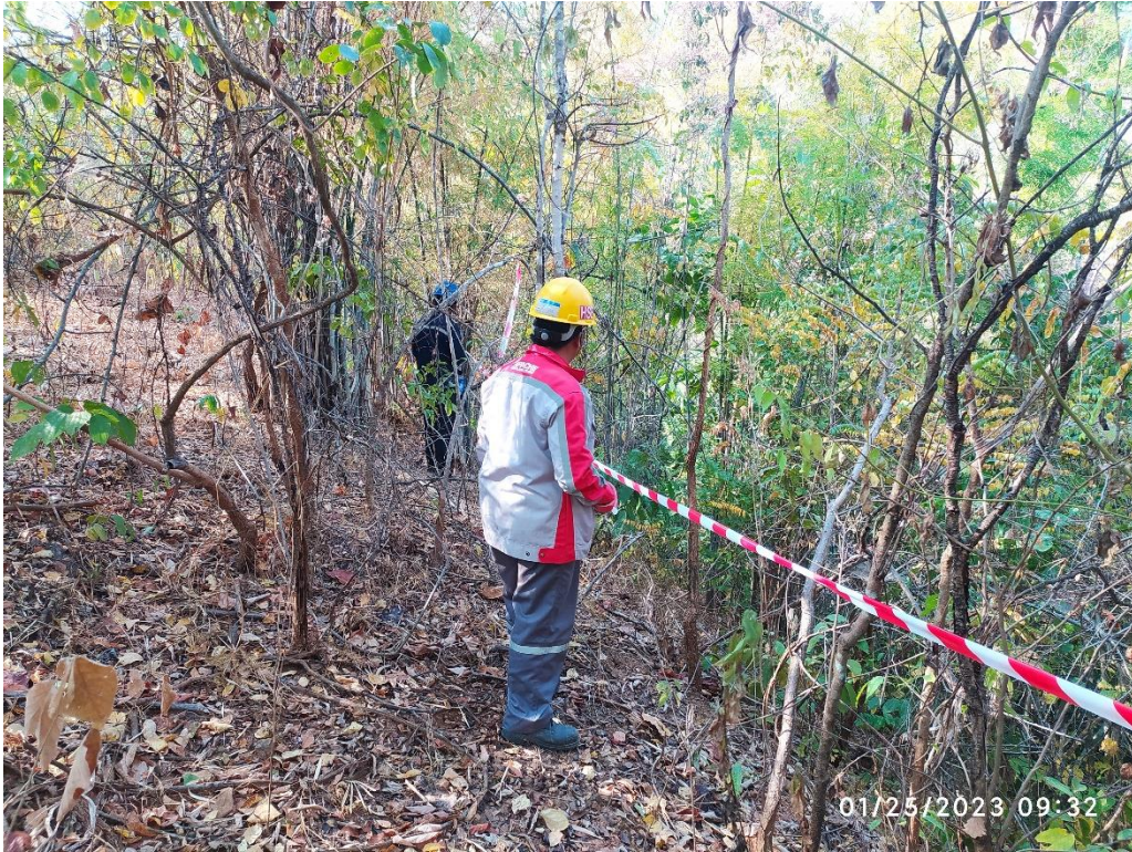
Photo of Land clearance at Red clay Quarry
