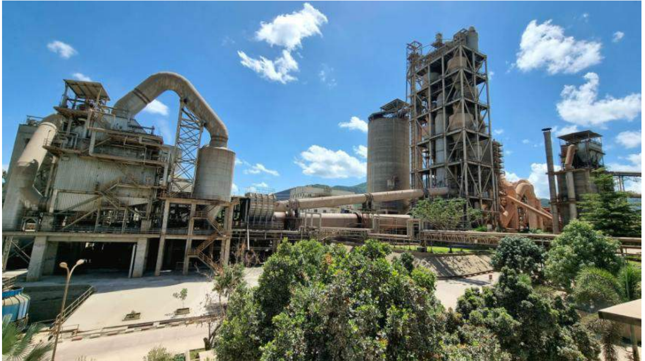
Figure 3. WHR System in STC Cement Plant
