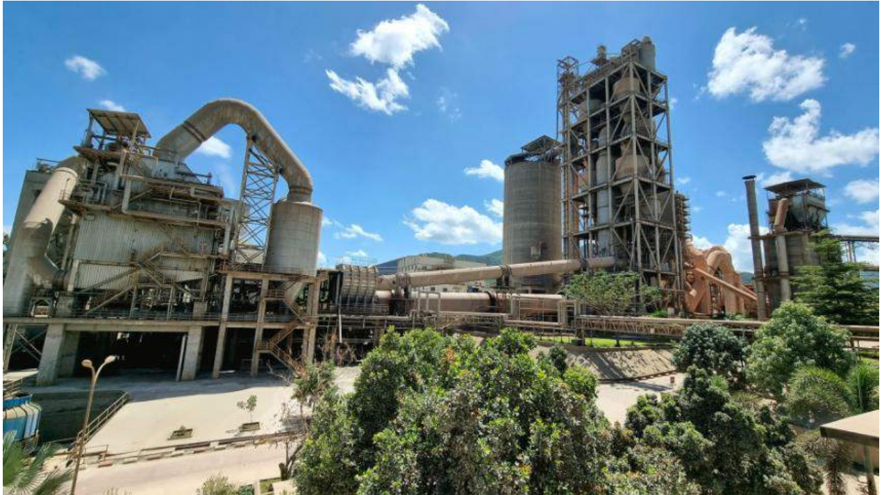
Figure 3. WHR System in STC Cement Plant
