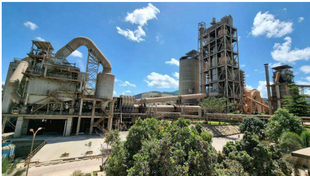
Figure – 3: WHR System in STC Cement Plant
